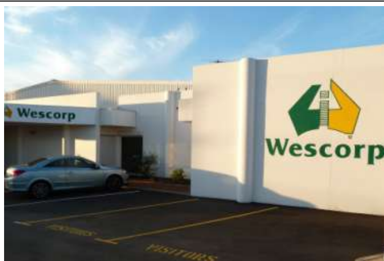
Wescorp's new premises in Canning Vale
